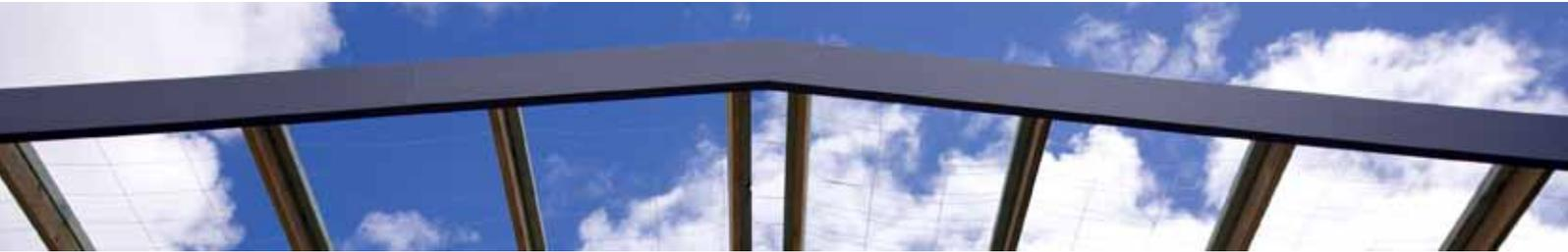
**AUSPINEblue** is Australian grown plantation pine framing that has been protected against termite and European House Borer (EHB) attack with long acting synthetic pyrethroid insecticides. It is dyed blue to make it easy to identify as being treated.
